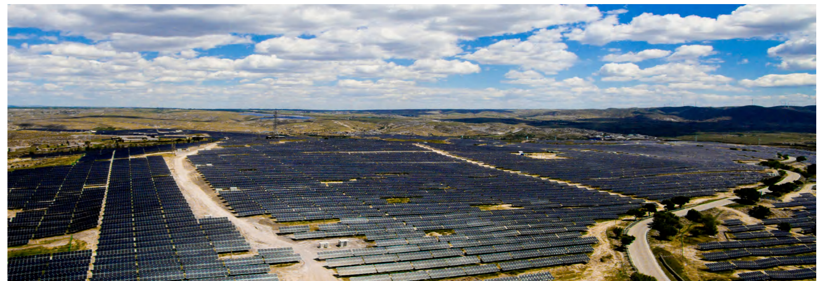
50 MW N-Type bifacial PV plant of national "Top Runner" advanced technology demonstration base in Datong, Shanxi Province, China
