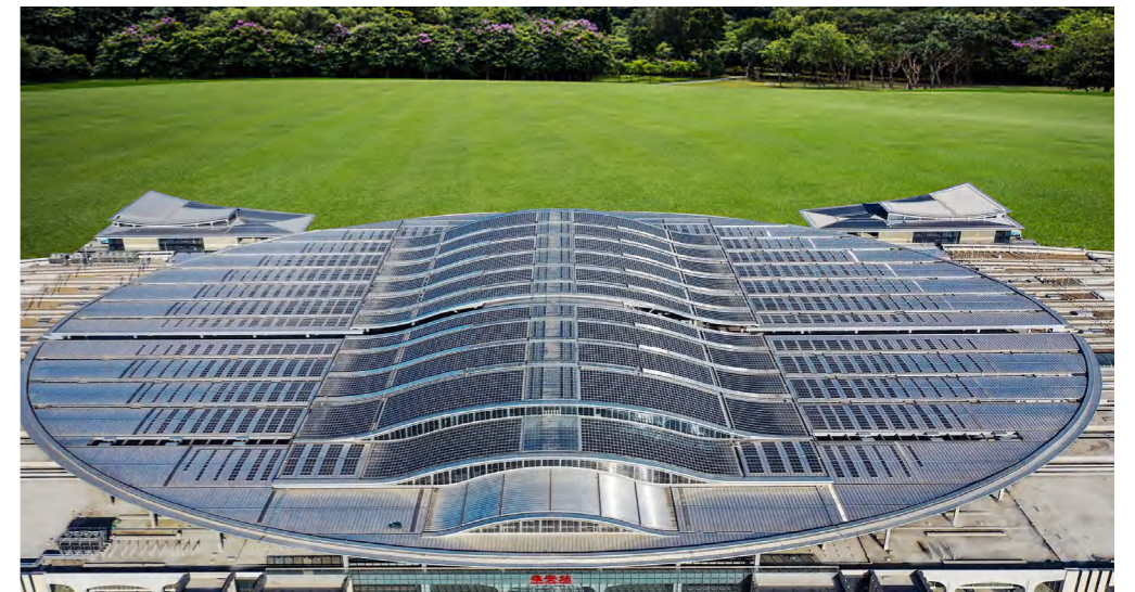
6 MW rooftop distributed plant at High-speed Railway Station in Xiongan, China
