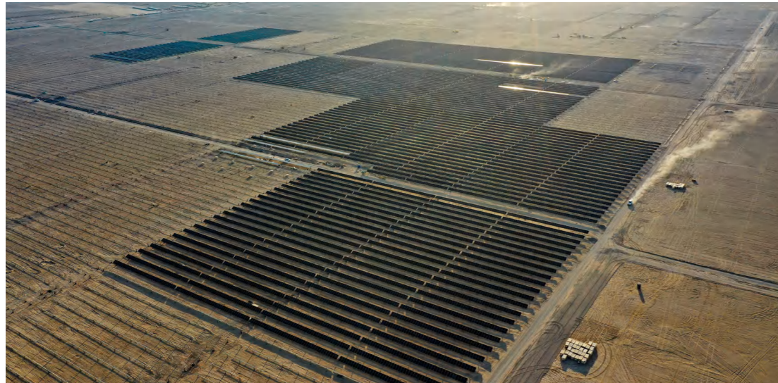
117 MW N-Type bifacial PV plant in Iberia, Oman
